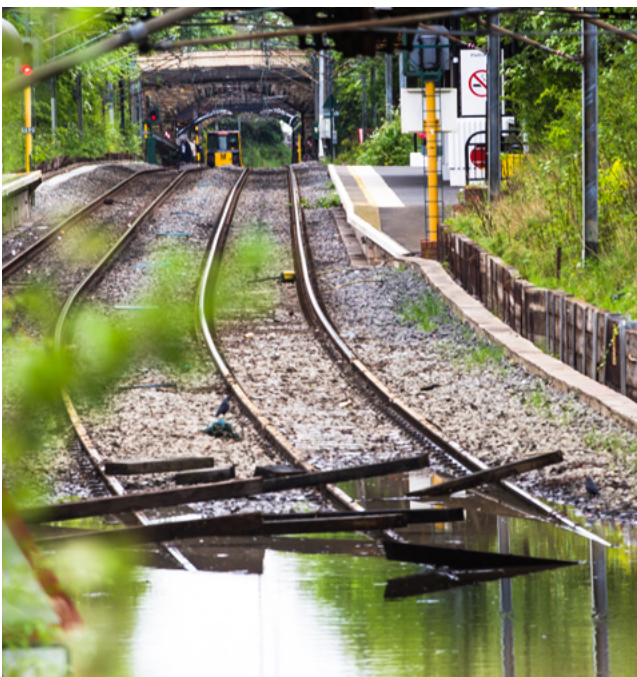
▶ A lack of drainage led to the flooding of the Tyne and Wear Metro in May 2017, forcing a 10 minute journey to take 1 hour.
