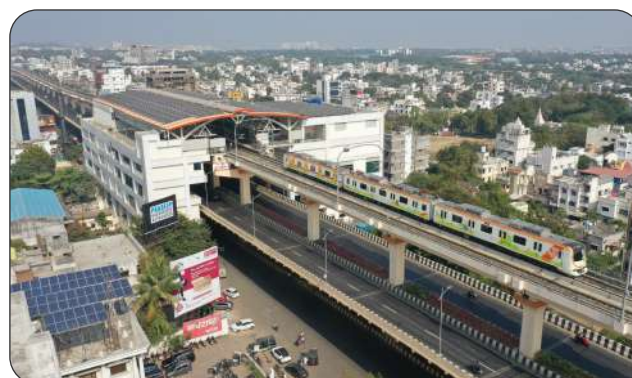
→ Aerial view of Nagpur Metro showing a stretch of the double-decker viaduct, supporting both a highway flyover and a metro rail on a single column ©Maha Metro
