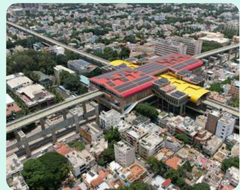
→ An interchange station of Bangalore Metro ©BMRCL
