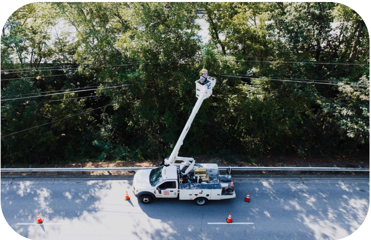
→ Electric wire repairs. Source: pexels.com | Kelly
